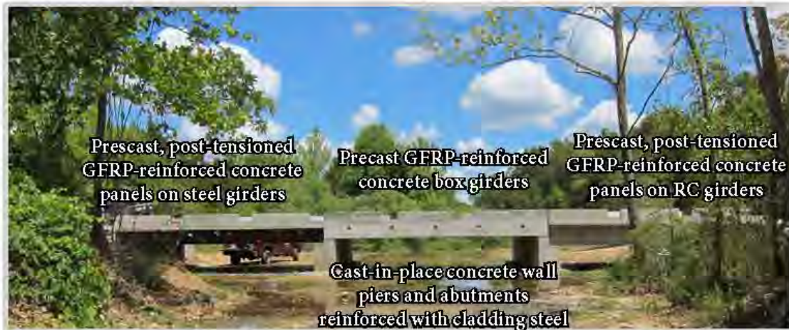
Figure 1. Complete three-span bridge over Arnault Branch, Washington County, MO
