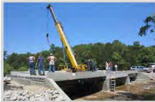
(a) Lift and placement of precast panel
