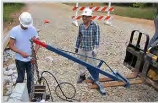
(b) Post tensioning of CFRP bars
